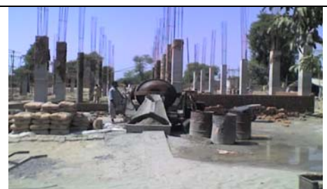
Construction Work of Arifwala Hospital is in Progress
