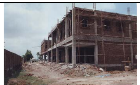
Construction Work of Pasrur Hospital is in Progress
