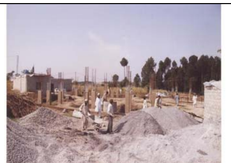
Construction Work of Mansehra Hospital is in Progress
